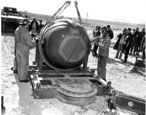
PLK 45-4 - 8Feb55 ESS weapon saddle with men attaching crane hooks.
